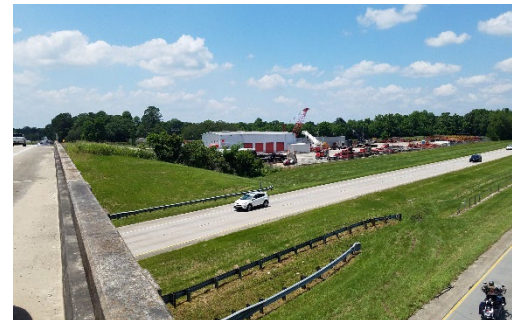
NW Quadrant, looking northwest from LA 74 overpass at ALL Crane Rental.
