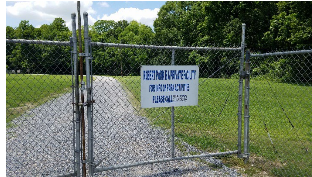
Secured entrance to Dutchtown Treatment Plant superfund hazardous waste site in NW quadrant,
